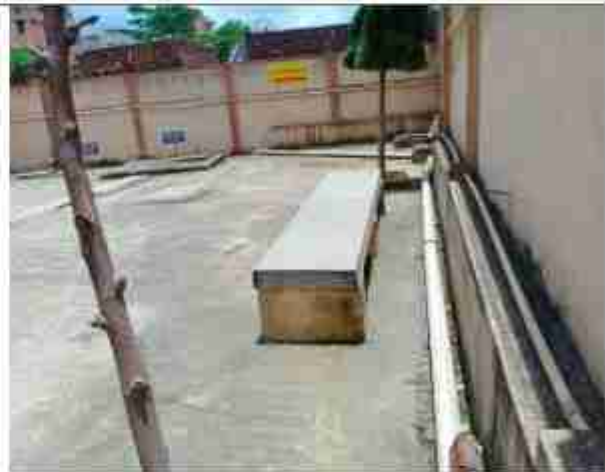
Rain water system with down comer and water collection circuits at Mango Campus
